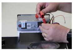
Connect the same red C connector into to the DOT loom red socket
